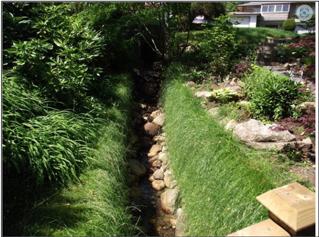
Figure 25 - Vegetated ditch lining system at acute changes in direction:
