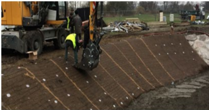
Figure 24 - Ditch lining materials for straight lengths
